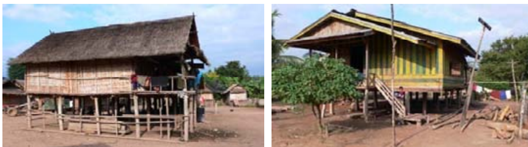
Figure 7-1 A and B: Existing Houses at Ban Xiengdet (A: bamboo and thatched roof; B: wood and corrugated iron roof)
