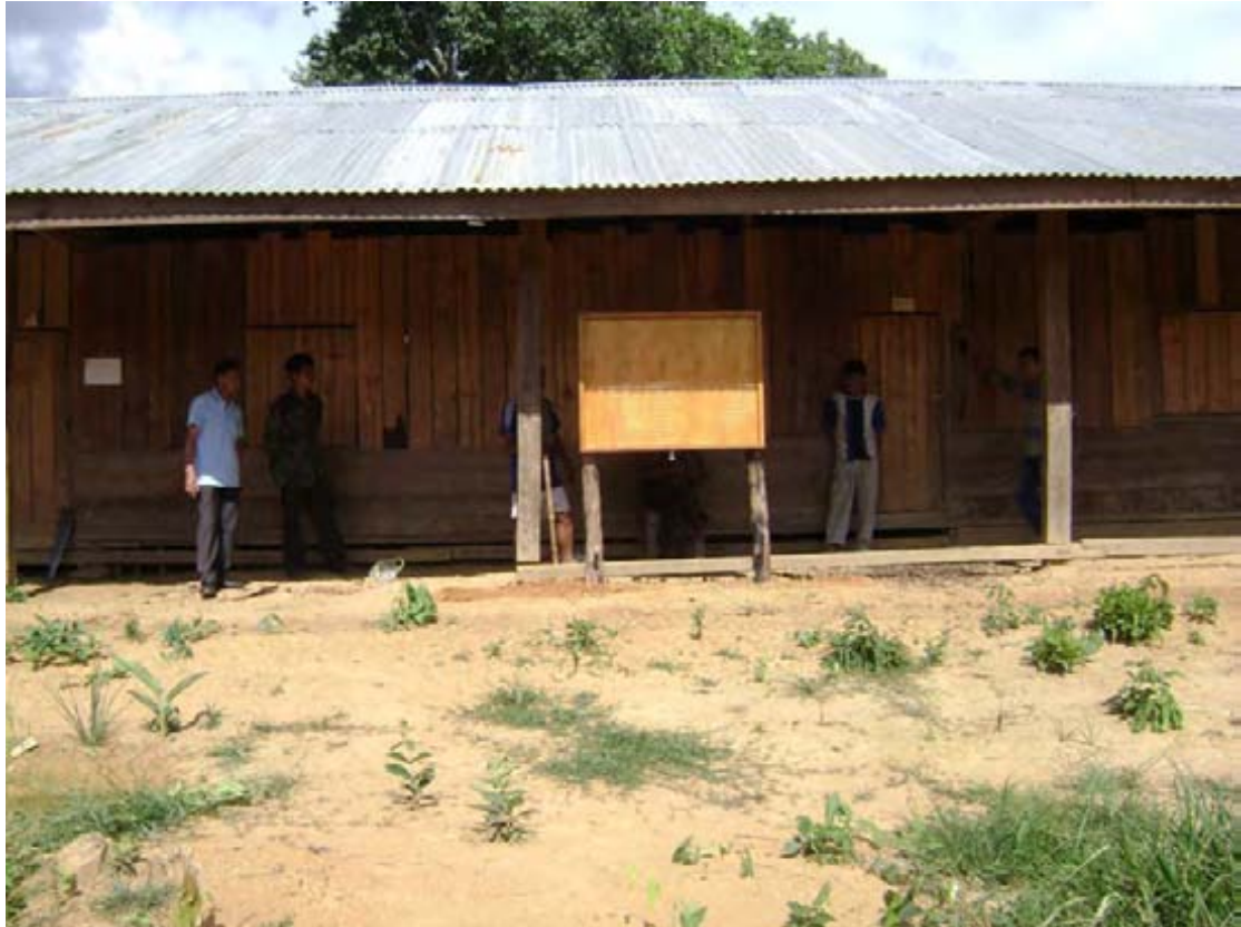
Installation of Notice Board at the New School, 23 June 2011
