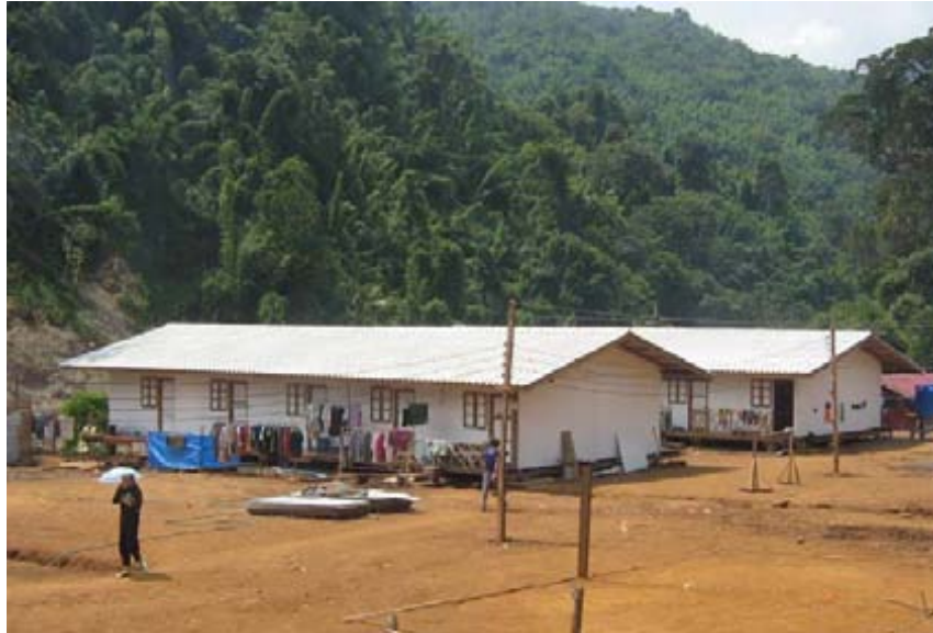
Figure 3: Work Camp at Power House (2007).
